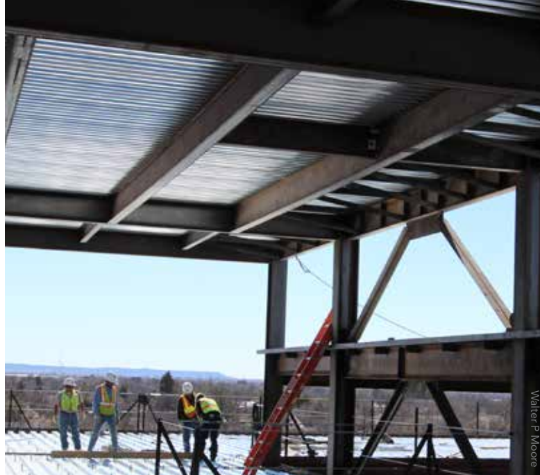
Steel bracing at the main roof and high roof.
