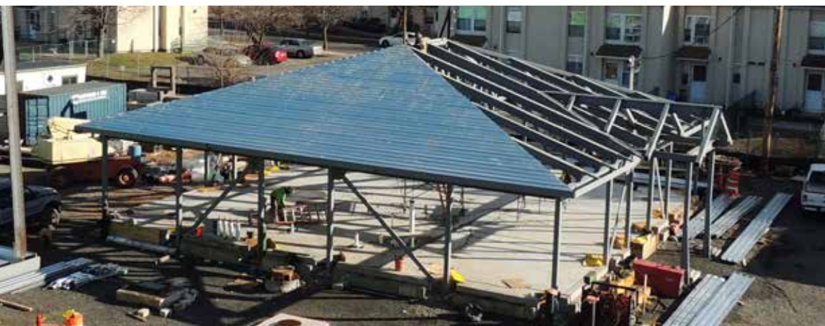
below: The framing for the smaller, administrative building consists of a combination of HSS sections and wide-flange beams, with the main lateral force-resisting system made of bracing built up in the perimeter walls.
