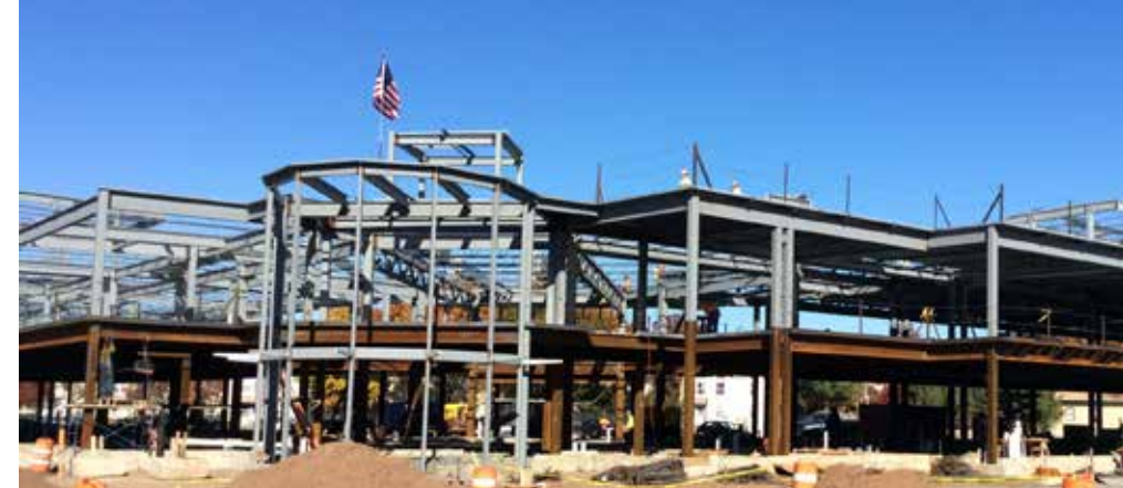
The main school building uses roughly 600 tons of structural steel framing.
