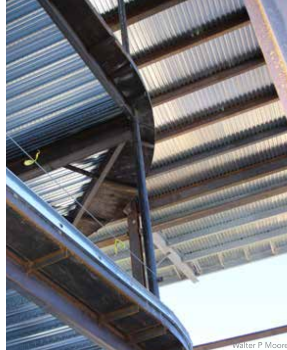
Framing for the pod assembly, which hangs from the ceiling in the atrium space.
