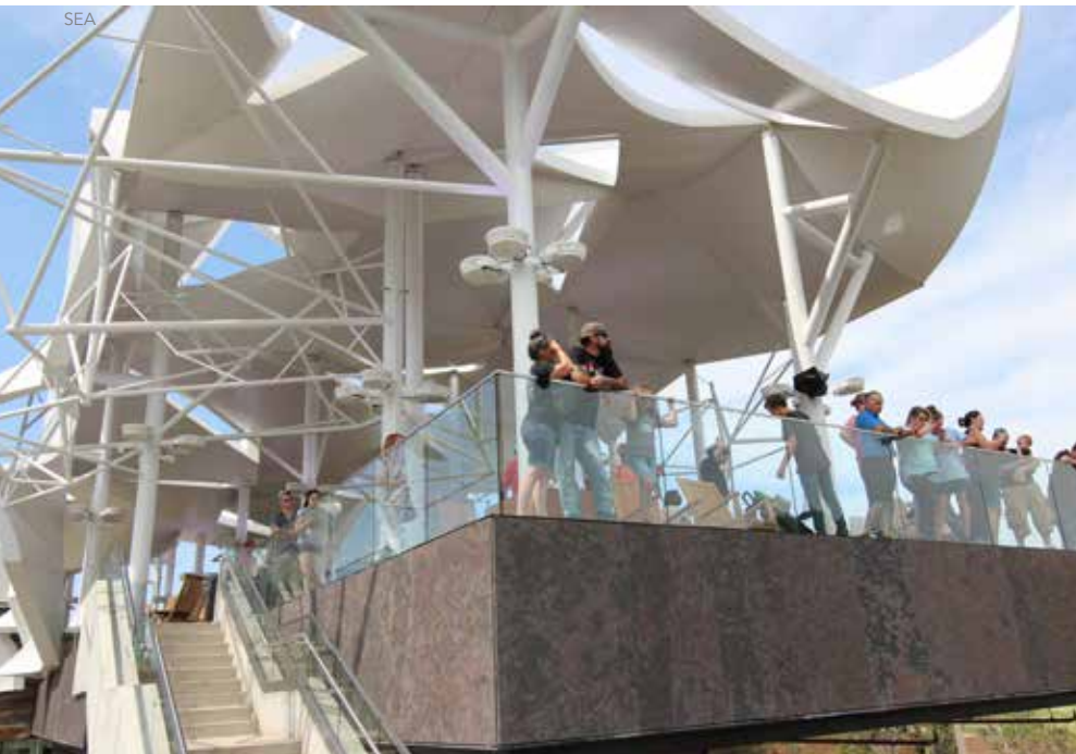
The centerpiece of the boathouse is a fiberglass canopy supported by HSS, that serves as the roof for the upper-most pavilion level.
