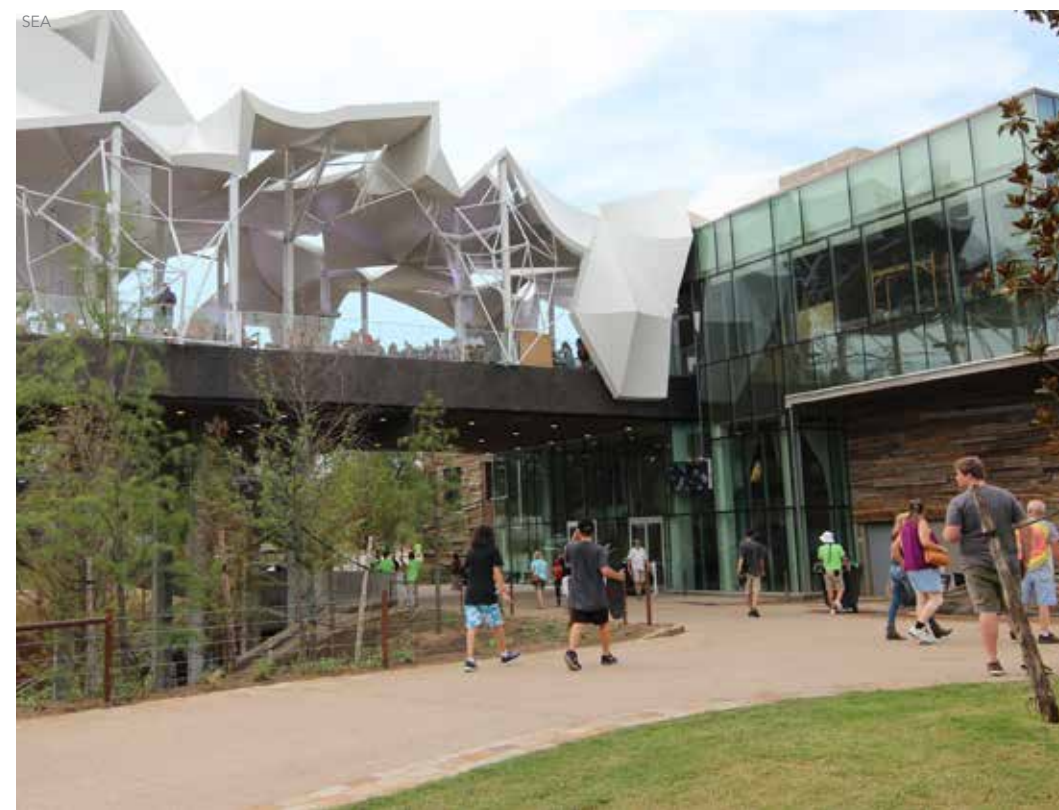
The centerpiece of the boathouse is a fiberglass canopy supported by HSS, that serves as the roof for the upper-most pavilion level.
