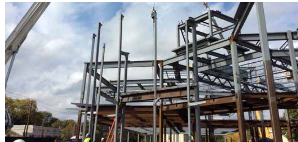
The main school building uses roughly 600 tons of structural steel framing.
