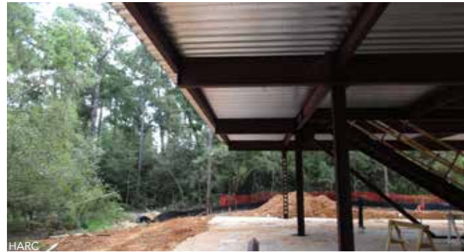
Wide-flange girders span the 62-ft direction of the building, and 24-ft composite steel beams span between the girders.
