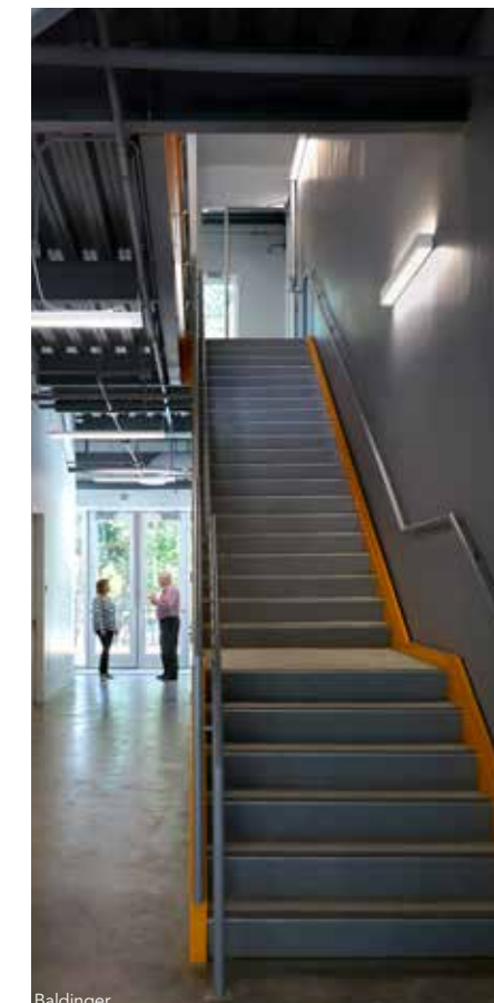
The steel-framed stairs, installed.
