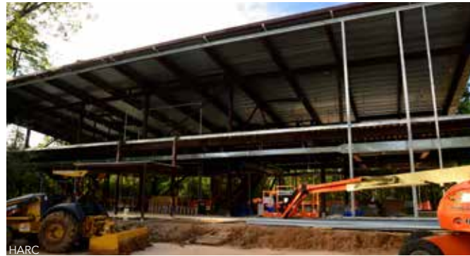
Wide-flange girders span the 62-ft direction of the building, and 24-ft composite steel beams span between the girders.
