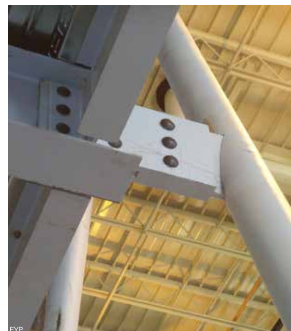
AESS connection of a floor beam to a truss diagonal.
